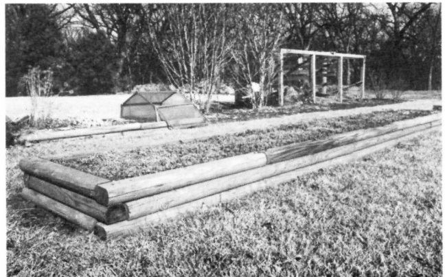
B. Reinforcing Rods Hold Timbers Together.
